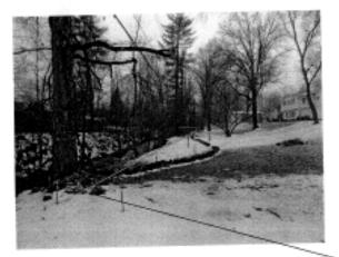
View looking South from North corner of Dr. to 1 red taped tree to be removed, yellow stake op of new modular block wall. All trees and invasive honeysuckle to be removed to left of red line, which is new wall line.
