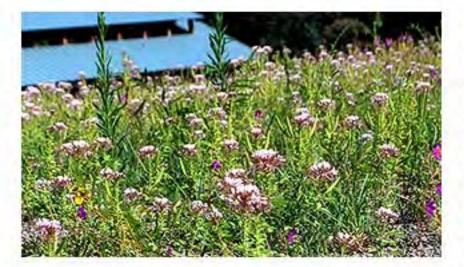
A green roof captures, slows down and reduces the quantity of rainfall before it enters the gutter. Green roofs also add energy savings by insulating the roof thus reducing heating and cooling costs. The existing roof must be reinforced to carry the additional weight load, anywhere from 15–30 lbs./sq. ft. or more depending on the depth of the soil. While installation of a green roof is initially more expensive than a conventional roof, a green roof has a
