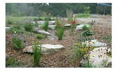
Bioswales can be constructed independent of a rain garden if circumstances don't allow for the installation of a rain garden (such as limited space or steep, narrow sites). In this case, they guide water to existing storm-water systems such as storm drains in roadways, etc.
