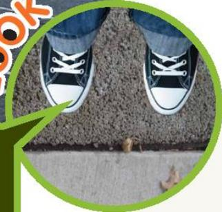
The concrete below your feet is no mistake! This odd looking surface is pervious concrete, designed specifically to absorb stormwater.
